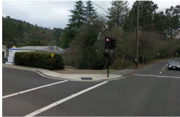
The existing curb extension southwest of the Risa Road/Mt. Diablo Boulevard/Village Center intersection creates a shorter crossing distance and a larger waiting area for pedestrians and bicyclists than a standard curb
