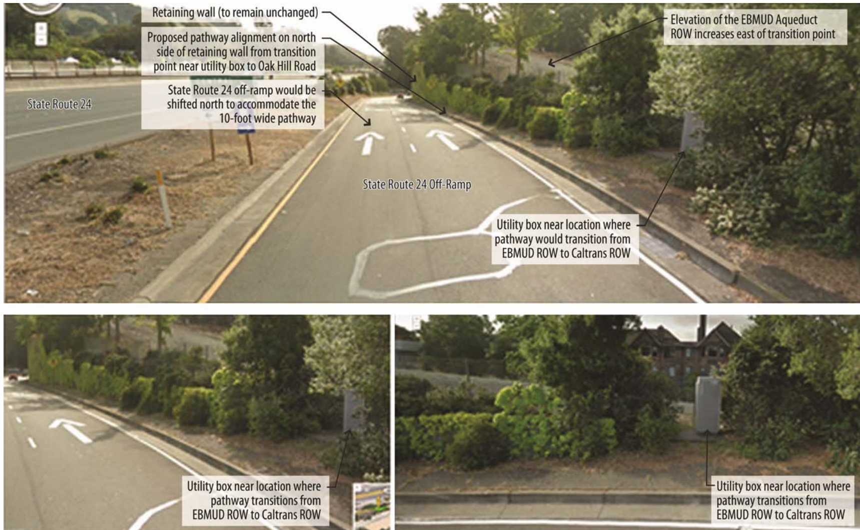
Figure 5-12: Transition point from EBMUD ROW to Caltrans ROW along the SR 24 eastbound off-ramp at Oak Hill Road
