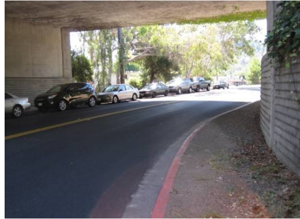
Looking south where Dolores Drive curves beneath SR 24, limiting stopping sight distances
