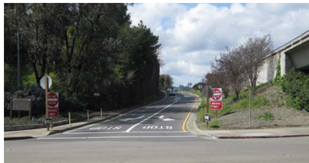
The SR 24 eastbound off-ramp at Oak Hill Road (looking west)
