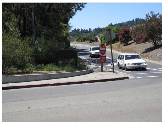
The SR 24 eastbound off-ramp at Oak Hill Road (looking west)
