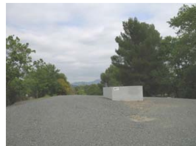
EBMUD Aqueduct Row Behind Terrace Way
