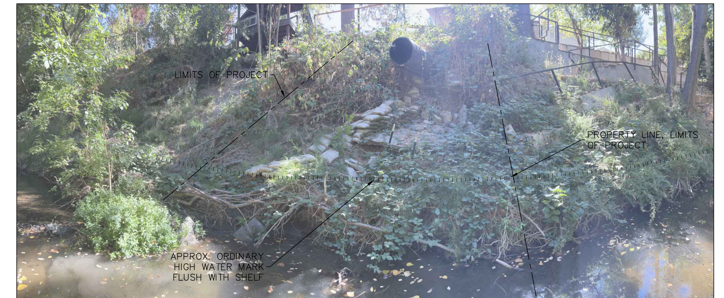
LAS TRAMPAS CREEK SOUTH BANK (OUTFALL)
