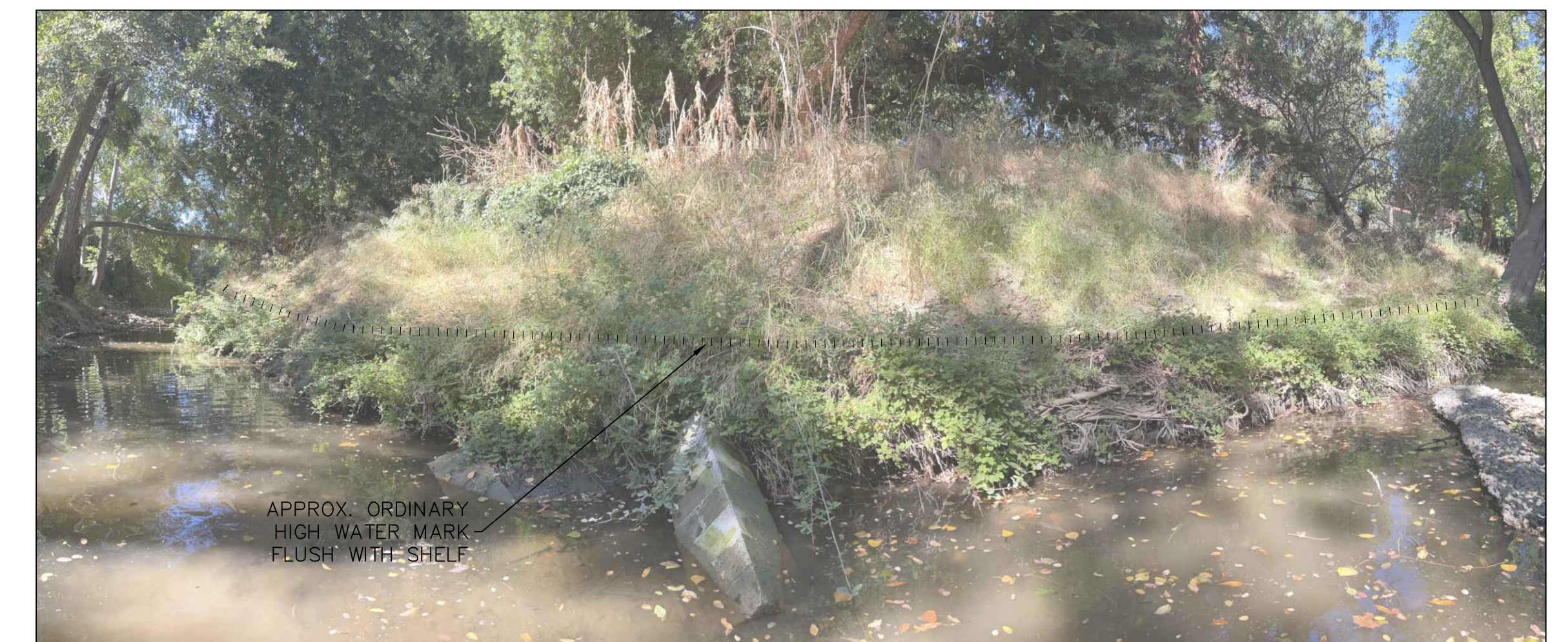
LAS TRAMPAS CREEK NORTH BANK (ACROSS FROM OUTFALL)
