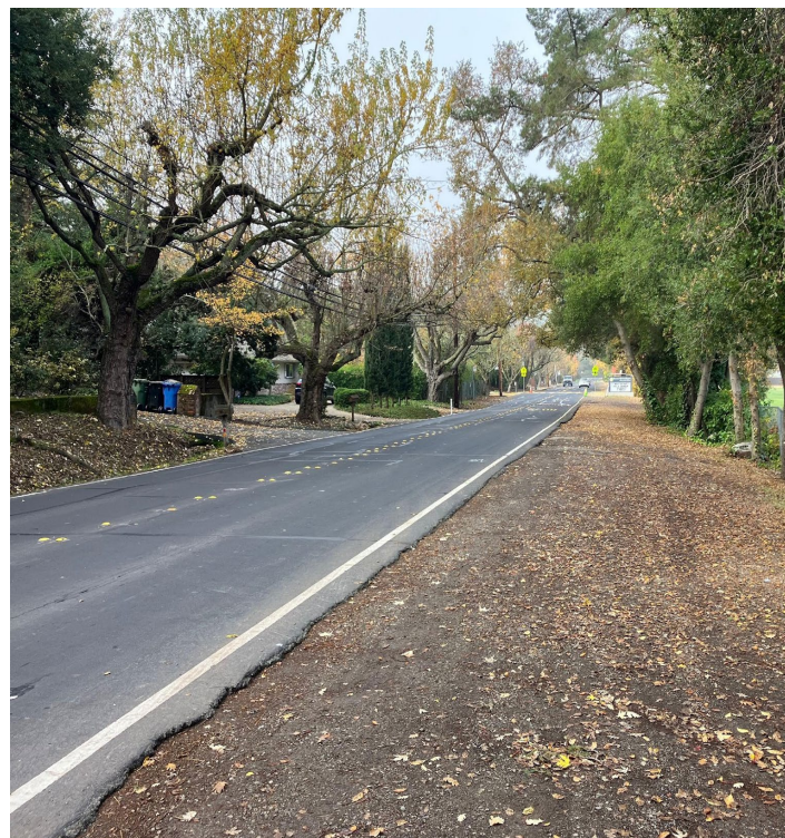
St. Mary's Road looking west towards existing drop-off area and Moraga Road
