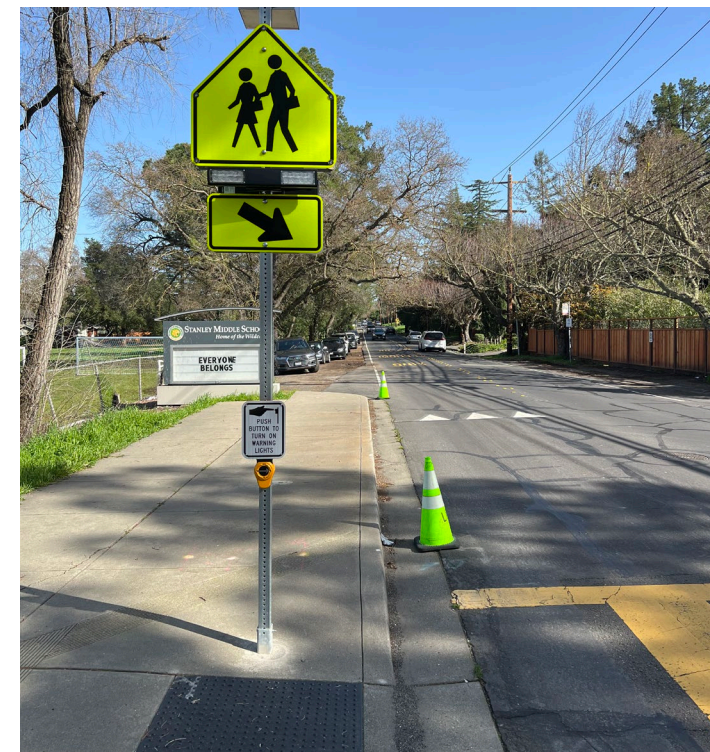
Existing End of Sidewalk
