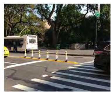
Hardened intersection centerline, concept graphic (Source: NYCDOT)
