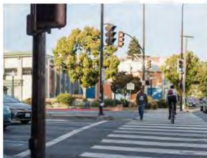
Continental crosswalk and stop bar (Source: Toole Design)
