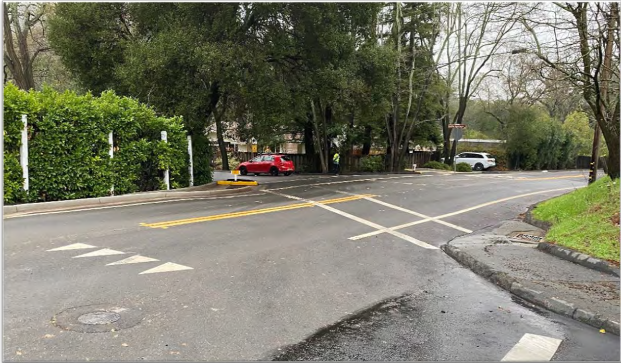
Figure 22. Crosswalk striping on Reliez Valley Road
