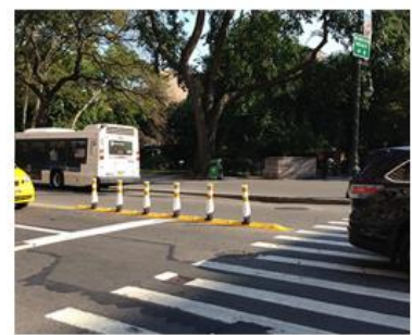
Hardened intersection centerline, concept graphic (Source: NYCDOT)
