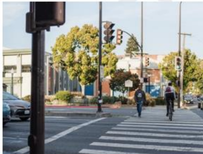
Continental crosswalk and stop bar (Source: Toole Design)
