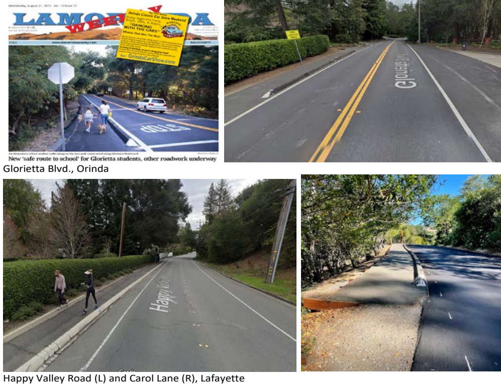
Figure 6. Examples of asphalt-berm-protected pathways (as presented by a community member)
