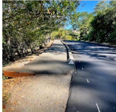
Figure 4. Examples of asphalt berm-protected pathways (as presented by community members)
