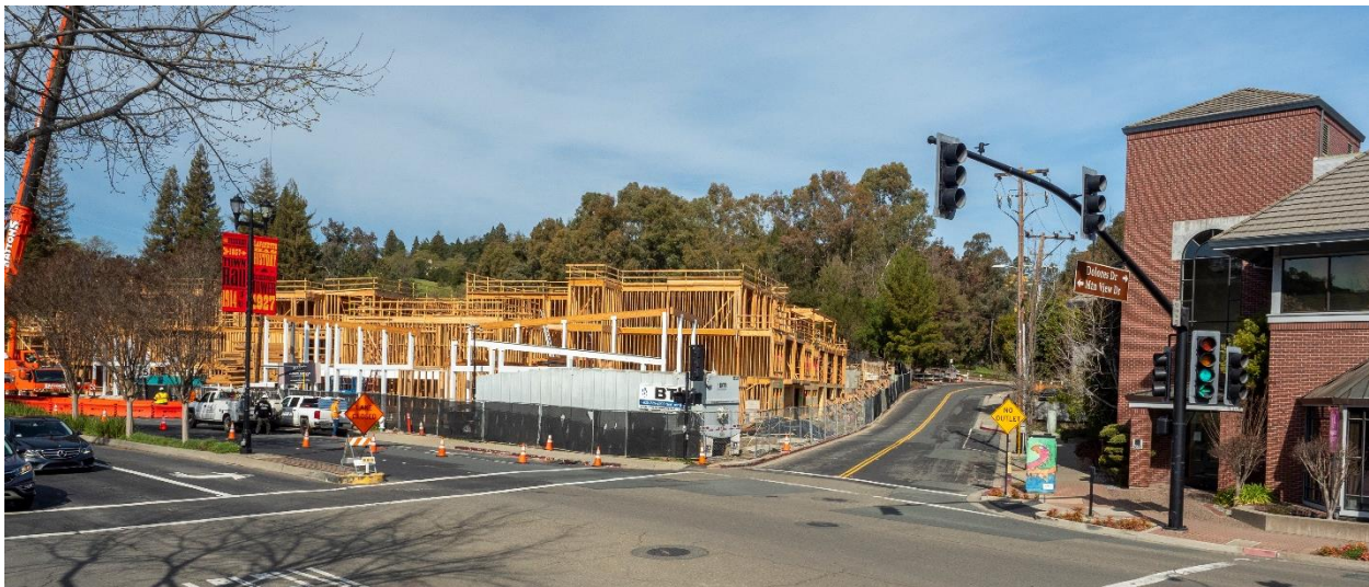
The Brant under construction in 2022.
