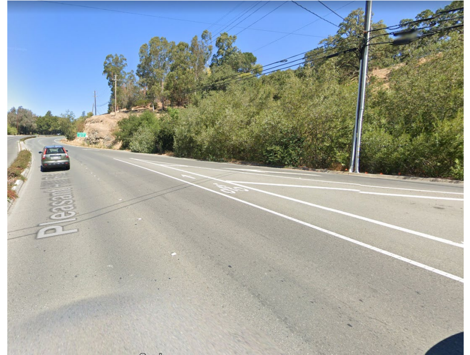
Source: Google Street View- Sept 2022 Slip lane merge with bicycle lane along Pleasant Hill Rd
