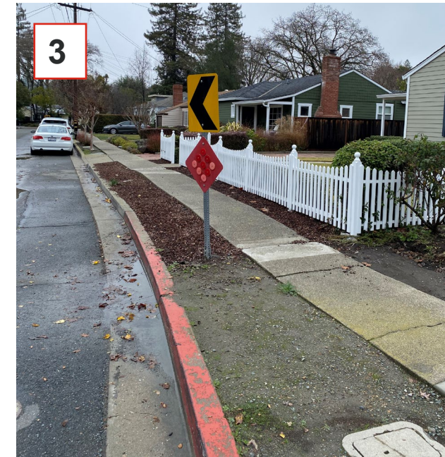
Source: Toole Design- Jan 2023 Narrow sidewalk along Moraga Blvd
