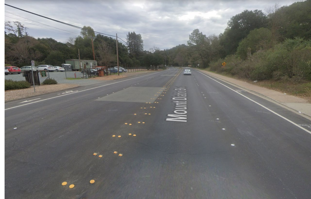
Source: Google Street View- Feb 2021 Typical cross section along Mt Diablo Blvd with narrow bike lanes and wide travel lanes
