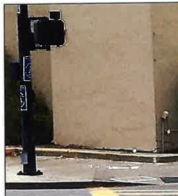
b) Single shared ped displays on SW and NE corners are off-axis to both served crosswalks
