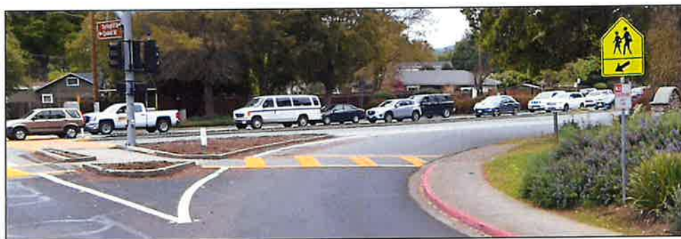
Figure 4-25: Eastbound-southbound slip lane crosswalk and warning sign
