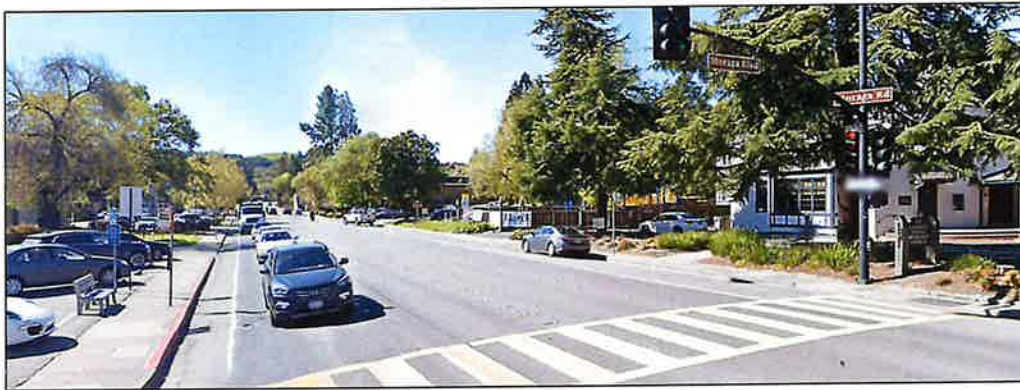
Figure 4-8: Moraga Road south crosswalk at Moraga Boulevard
