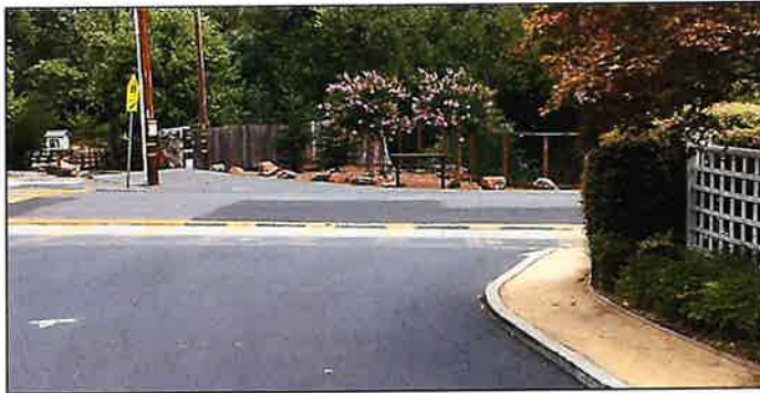
c) San Reliez NB approach – STOP sign hidden by tree
