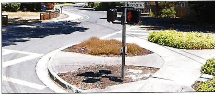
a) Existing button location
