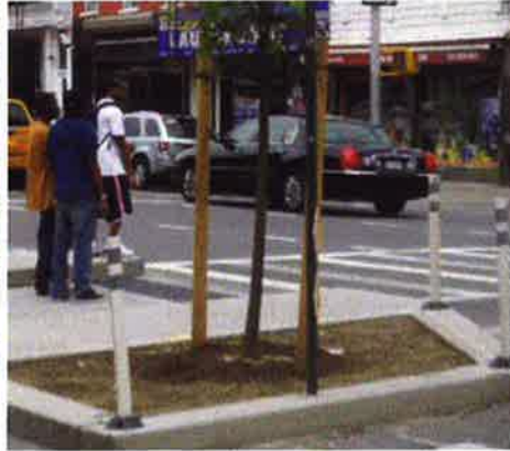
Figure 8. Flexible bollards on pedestrian island (New York, NY) Source: NACTO
