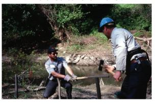
Installing willow posts with a mallet to control stream bank erosion is an easy solution for property owners
