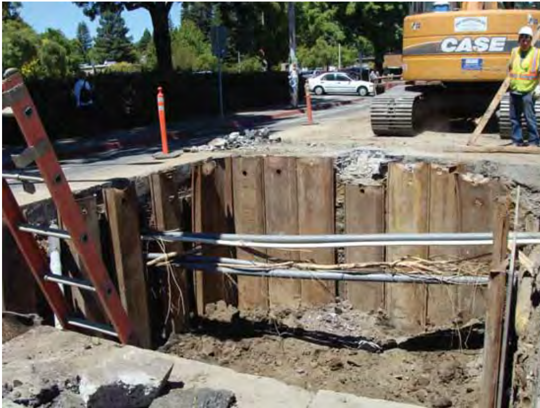
Figure 3. Tree roots can proliferate in utility trenches. Here, lateral roots of ash ( Fraxinus sp.) have grown along buried utility lines. Photo by K. S. Jones.
