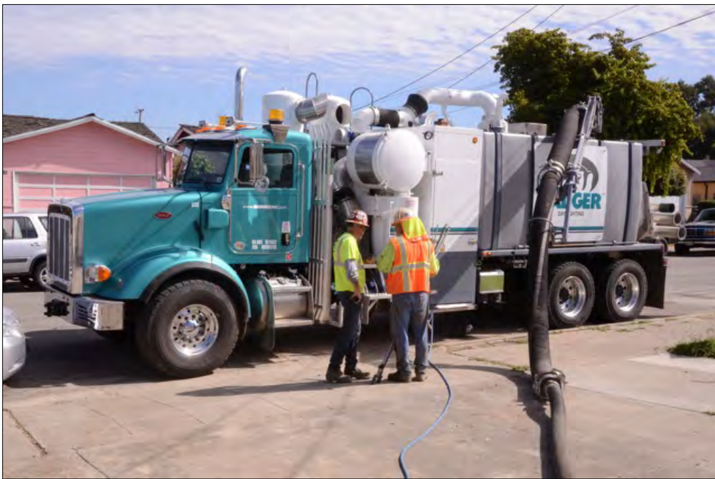
Figure 1. A typical Hydro-Vac truck.
