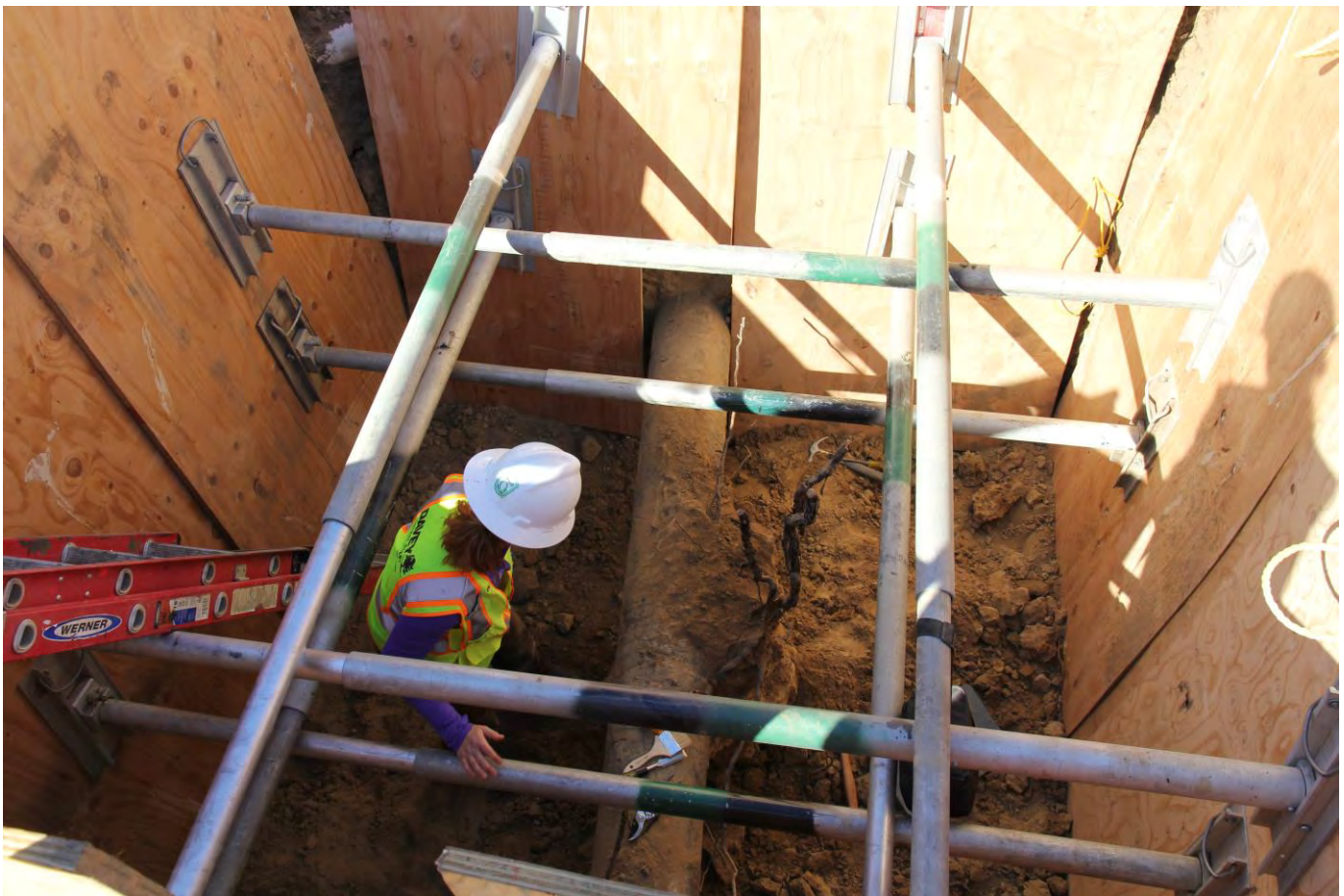
Figure 15. The roots from the Zinfandel grape vine at the pipeline level.
