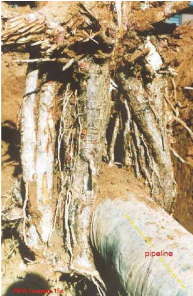
Figure 10. Oblique roots of a tree planted in proximity to a buried pipeline have come in contact with the pipe coating, causing damage. Photo from PIPA (2010).
