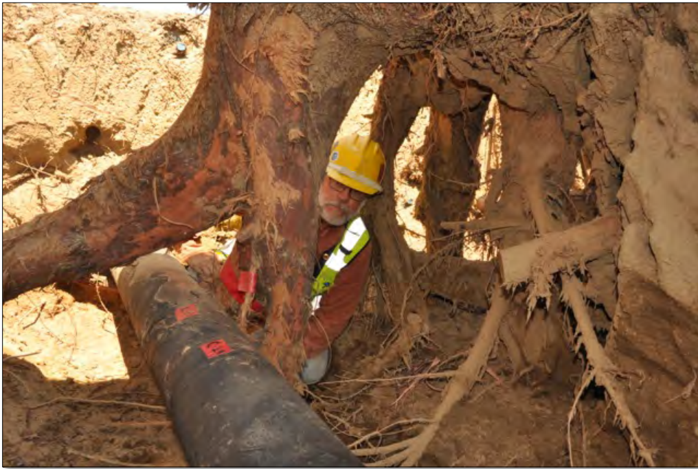
Figure 14. Eucalyptus root system in un-irrigated soils at dig site RWVIM-126-13
