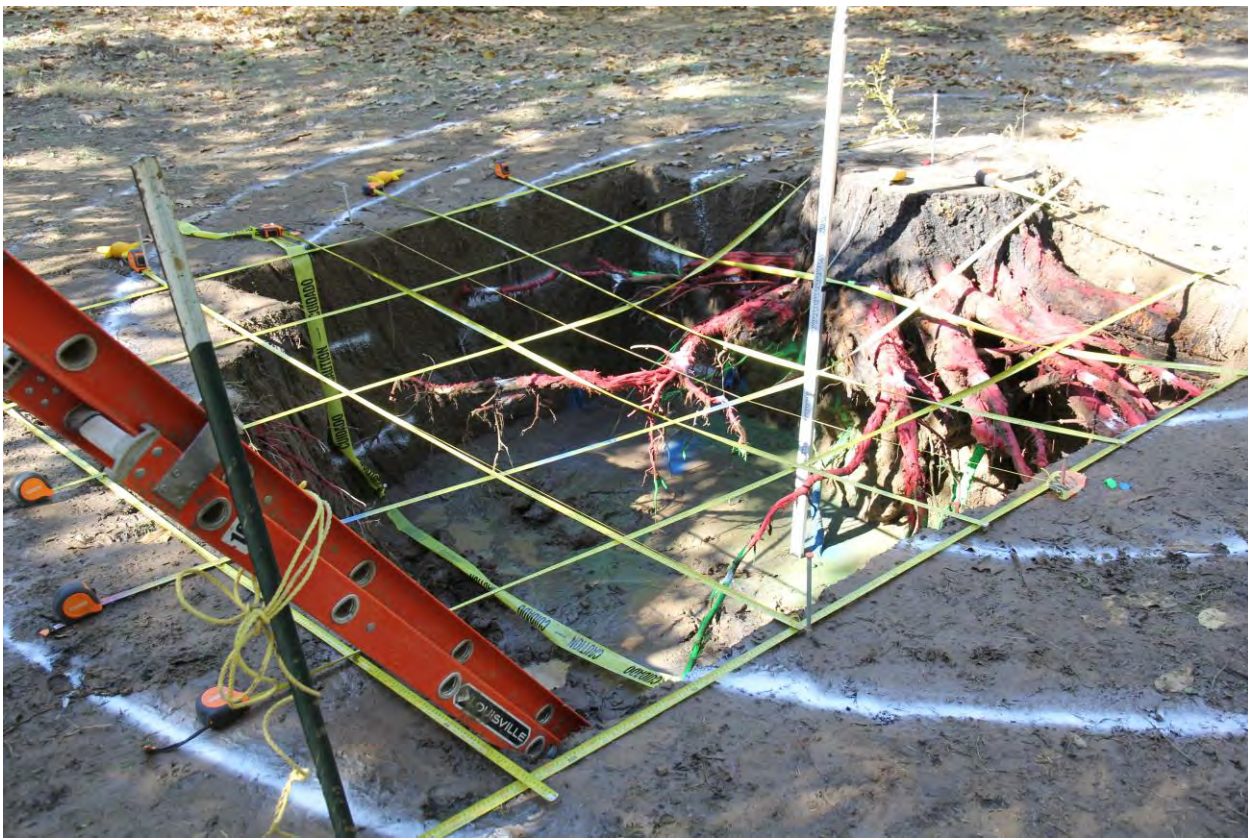
Figure 11. The walnut tree stump at Lockeford excavated to a depth of 4'. The pipeline is below the yellow "caution" tape on the bottom of the pit.
