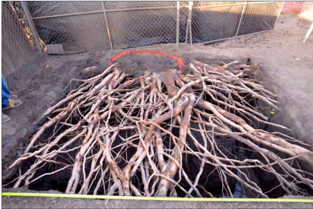
Figure 4. A lateral root system at 153-1.
