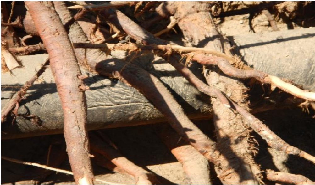
Figure 3. RWVIM-107-13 (Weber Lane) (CTE coating damage)
