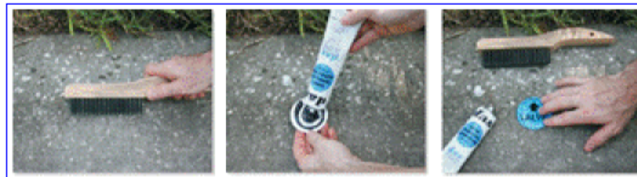
Figure 5. Curb Indicator Installation
