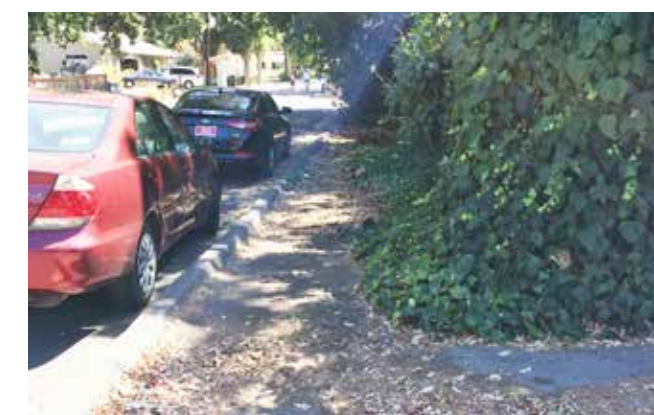
2nd Street lacks a sidewalk.
