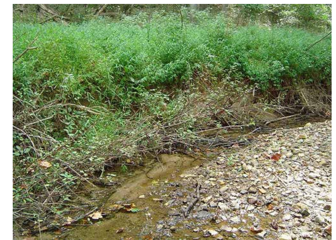
Brush layering for erosion control
