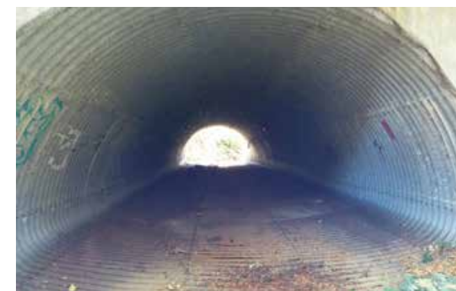
Culvert beneath church parking lot
