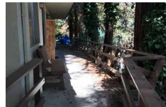
Pedestrian walk adjacent to creek is unused.
