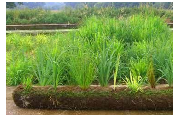
Biodegradable coir roll erosion control
