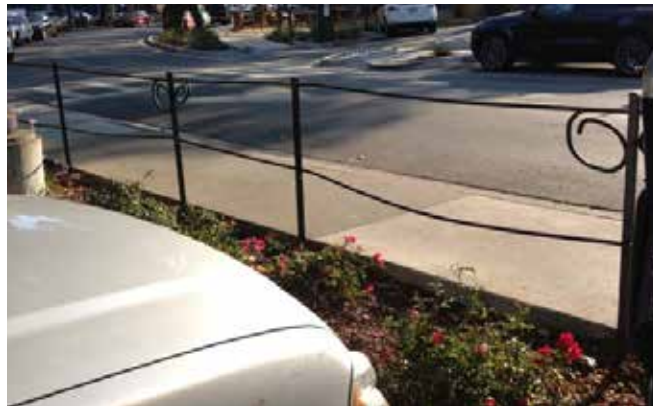
Fence / railing treatments
