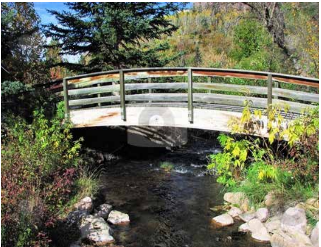
Example of bridge over creek
