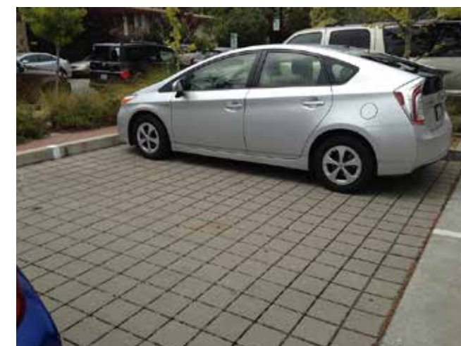
Pervious pavers in parking lot
