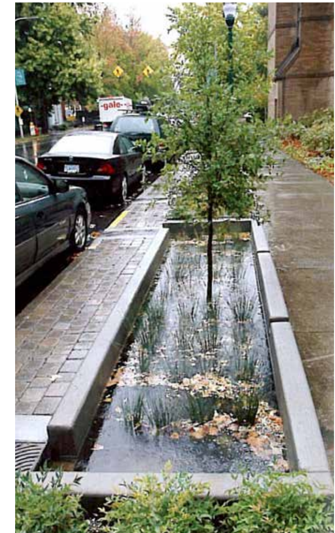
Rain garden in sidewalk area
