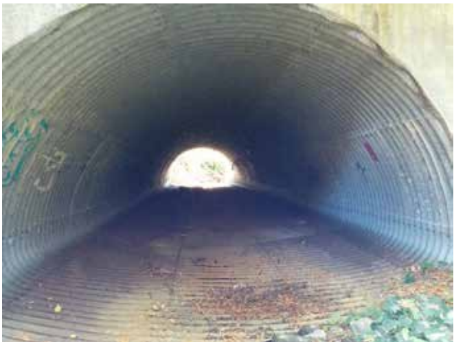
Creek at existing culvert
