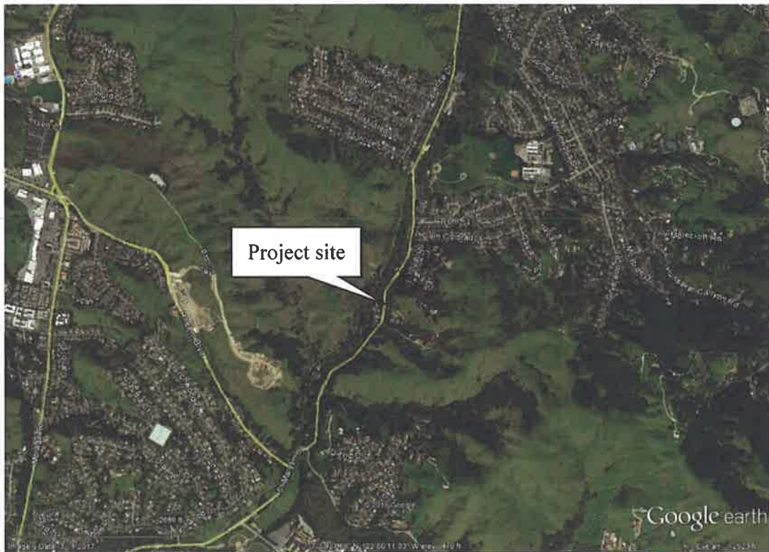
Figure 1: Vicinity Map and Aerial View of St. Mary's Road Slide Project Site
