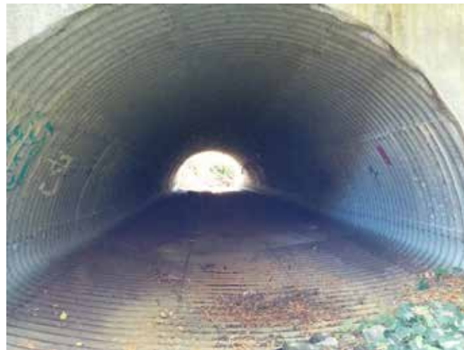
Creek at existing culvert
