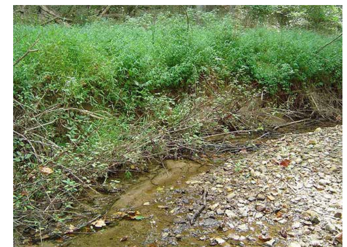
Brush layering for erosion control
