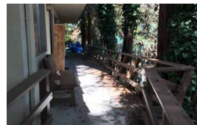
Pedestrian walk adjacent to creek is unused.
