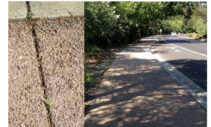
Pervious concrete sidewalk along Mt. Diablo Blvd.
