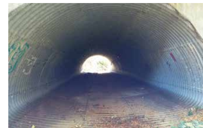
Culvert beneath church parking lot
