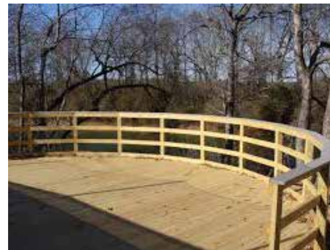
Creek overlooks encouraged, subject to determinations regarding bank stability, erosion, and water quality
