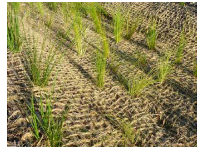
Biodegradable geotextile erosion control
