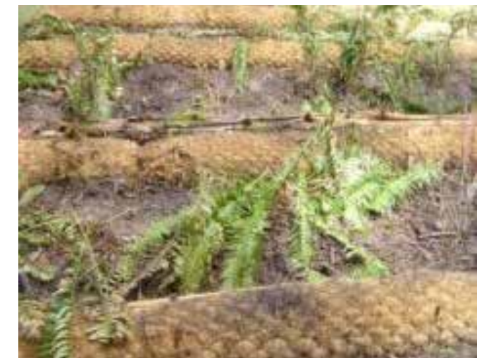
Biodegradable coir roll erosion control
