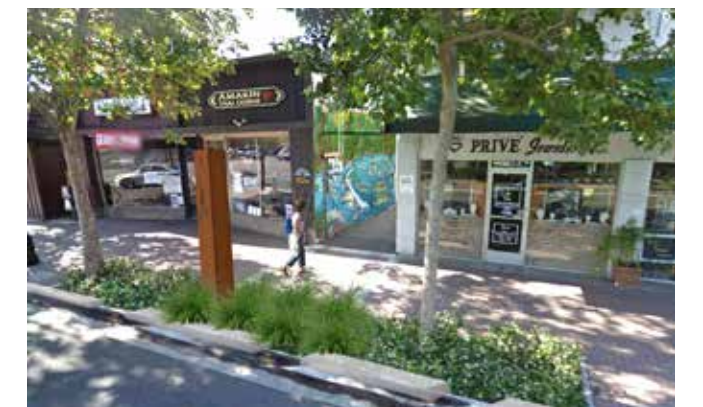
Proposed rain gardens and creek icon along Mt. Diablo Blvd. are public improvements; conversion of driveway to pedestrian access would be a private improvement
