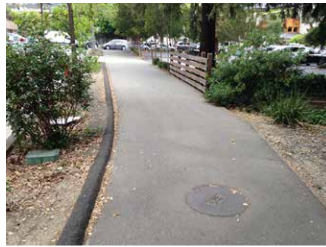
First Street, east side - opportunity to convert existing planting area to rain garden
