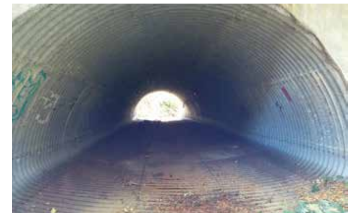
Culvert beneath church parking lot
