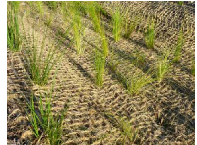
Biodegradable geotextile erosion control
