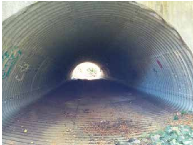
Creek at existing culvert
