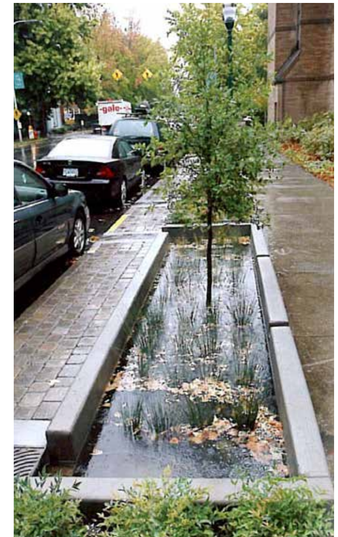
Rain garden in sidewalk area
