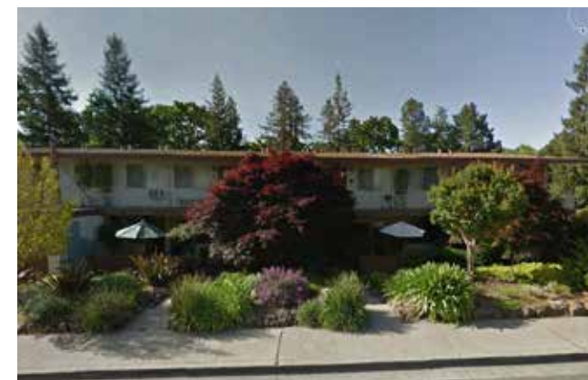
Treetops indicate creek corridor behind building
