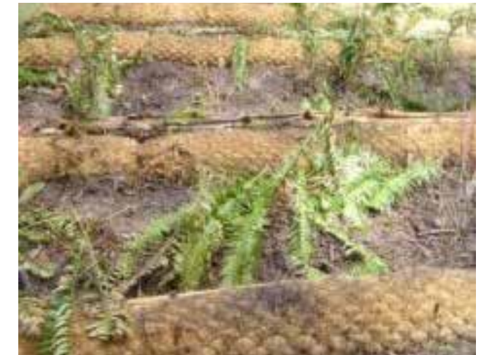
Biodegradable coir roll erosion control
