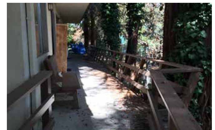
Pedestrian walk adjacent to creek is unused.
