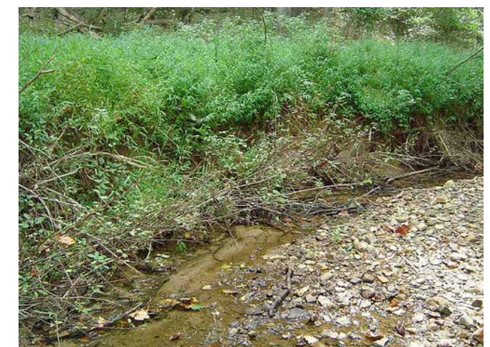
Brush layering for erosion control
