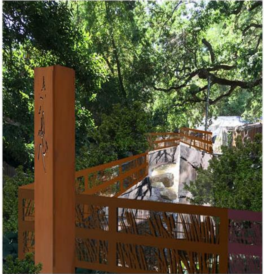
LOOKING EAST ALONG CONCRETE CHANNEL
