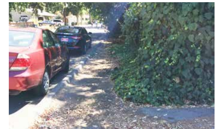
2nd Street lacks a sidewalk.
