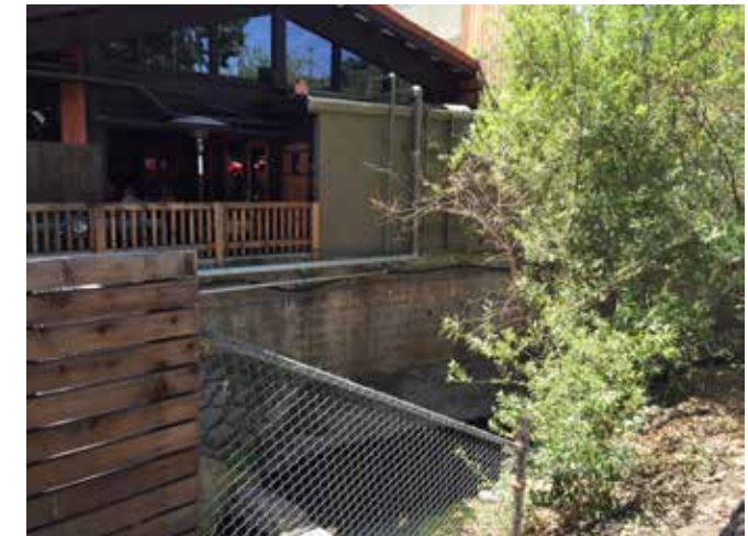
The foundation wall of the Cooperage could be an opportunity for a creek mural.
