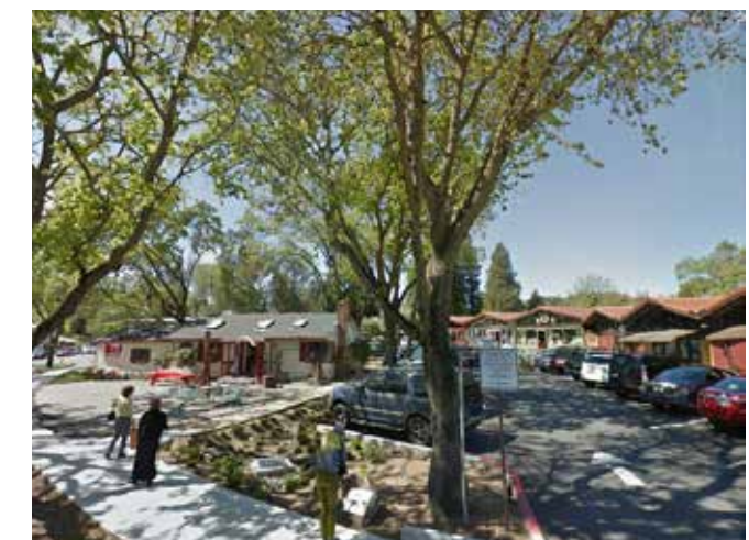
Bioretention area located in the parking area across from The Cooperage American Grill.
