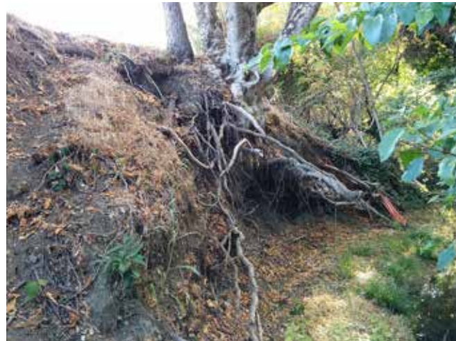
Exposed tree roots at West Reach
