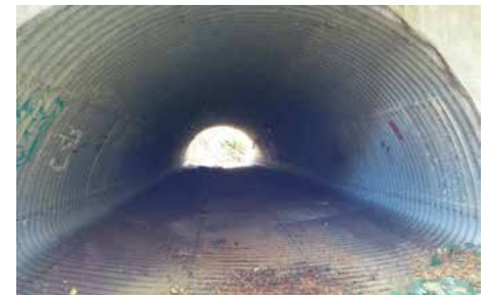
Culvert beneath church parking lot
