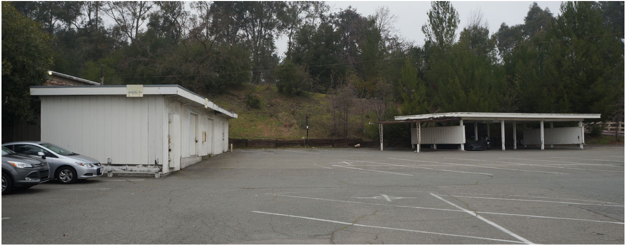
View of the northern portion of the parcel numbered 3666, showing the storage building (Structure 2) at the left and the carport (Structure 3) at the right.
