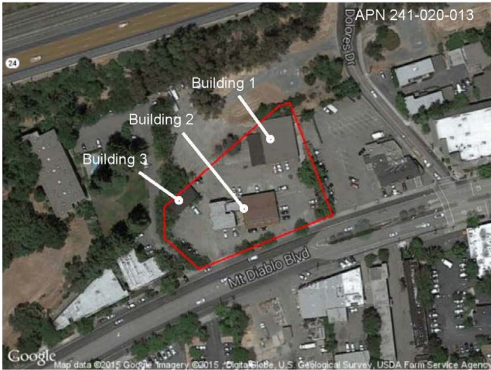
View of APN 241-020-013 / 3670, 3674-3678/3678a/3680 and 3684 Mt. Diablo Boulevard, showing the three buildings on the site. (Contra County Tax Assessor.)
