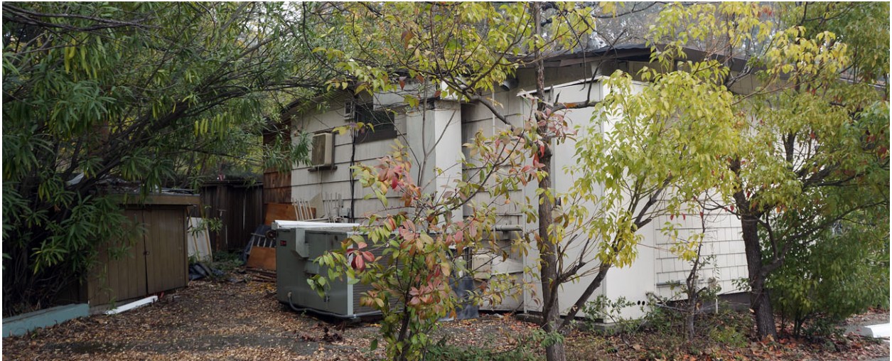
View of the north wall of Building 3, looking southeast.
