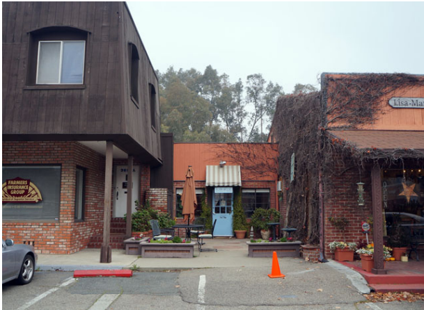
View of 3678a (second section of Building 1) which is recessed from back between 3674-78 (first section at the right) and 3680 Mt. Diablo Boulevard (third section at the left).
