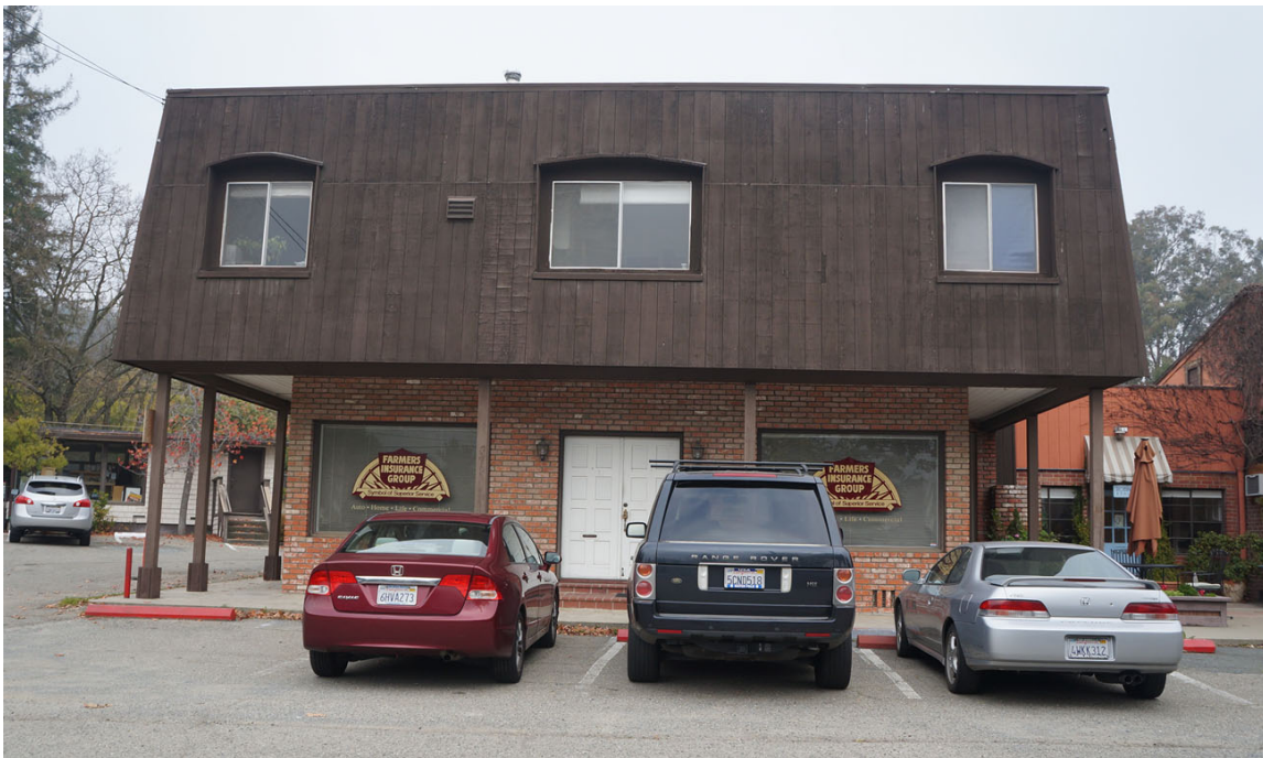
View of the south exterior wall of 3680 Mt. Diablo Boulevard, with 3678a at right.
