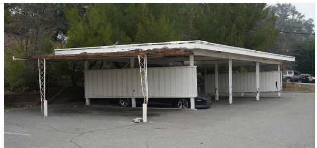
View of the south side of the carport (Structure 3), looking northeast.
