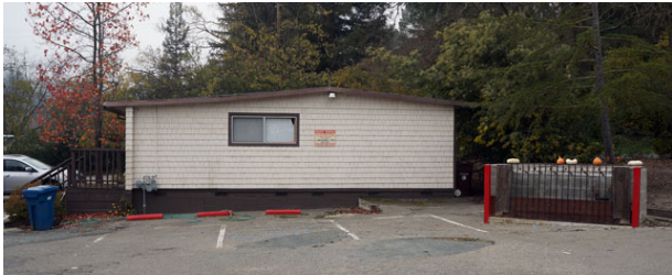
View of the east exterior wall of Building 3.
