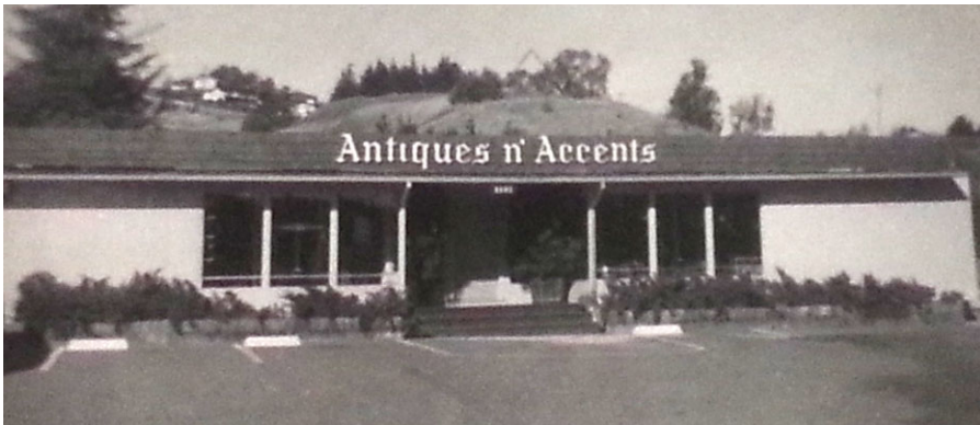
Historic view of the south wall of Building 3 at 3684 Mt. Diablo Boulevard. (Contra Costa County Tax Assessor, no date.)
