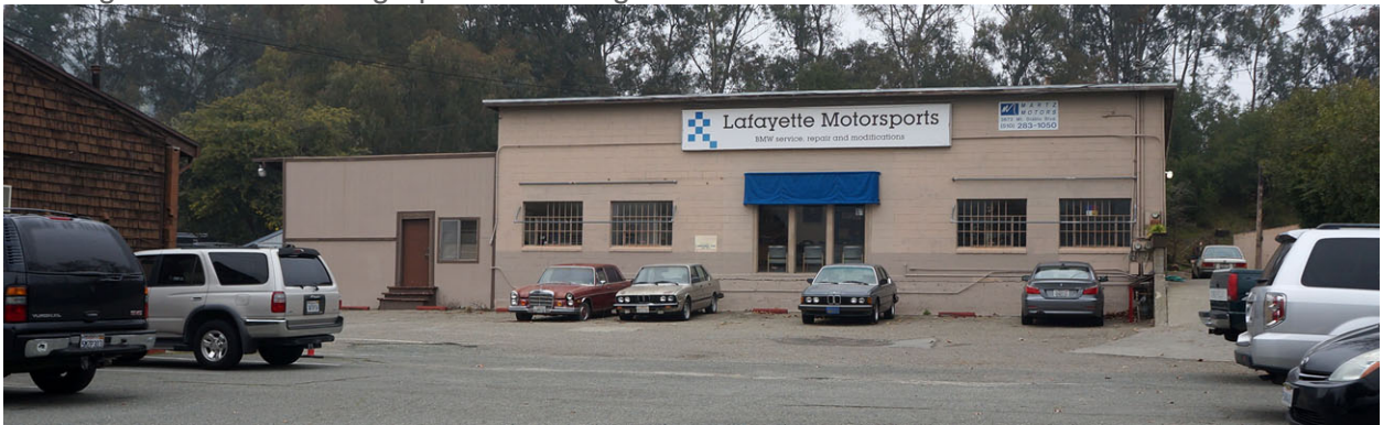
View of the south exterior wall of Building 1, looking north.
