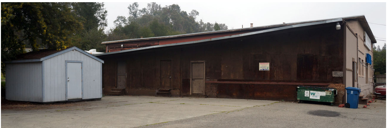
View of the south side of the west exterior wall of Building 1, looking northeast.
