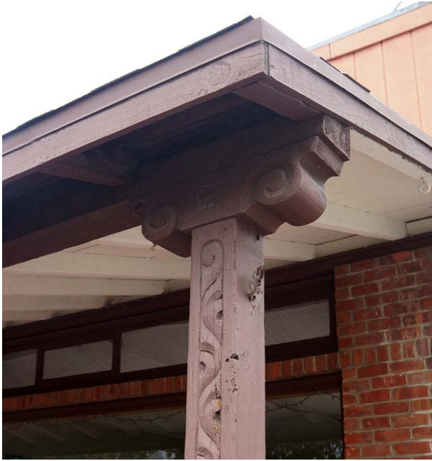
Detail of ornamental porch cushion capital and post.
