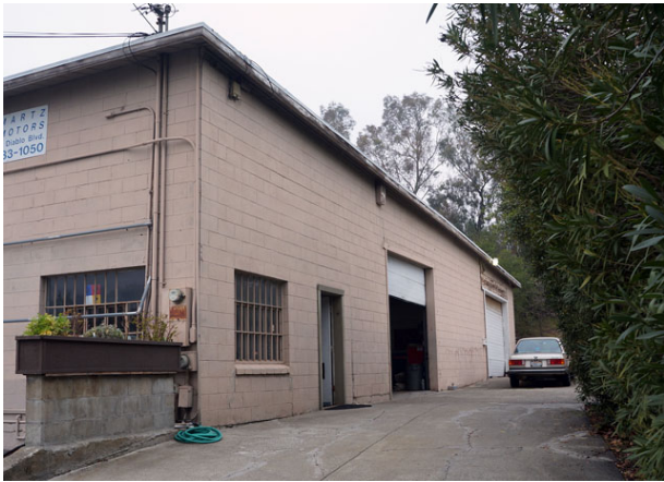
View of the of the east exterior wall of Building 1, looking north.
