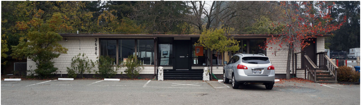
View of the south wall of Building 3, looking north.
