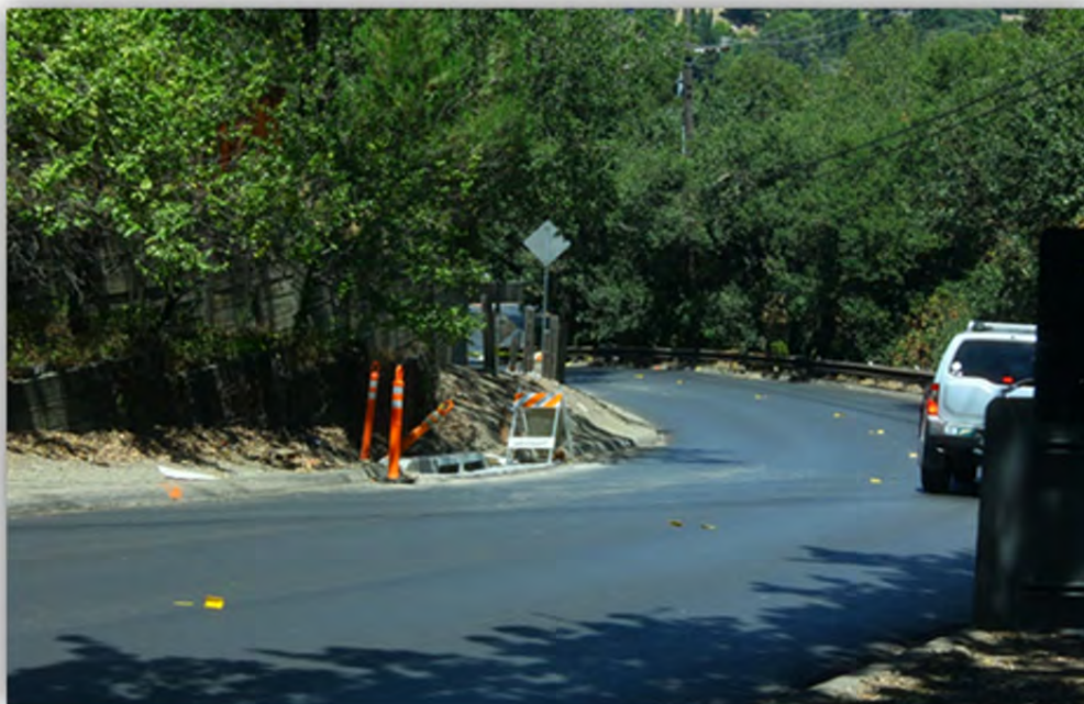
Figure 28: Sight Distance View from Richelle Court #2
