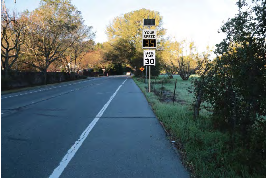
Figure 15: Westbound Olympic Boulevard – Proposed Speed Feedback Sign
