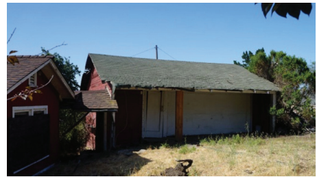
Garage, looking south. Portion of house is visible at left.
