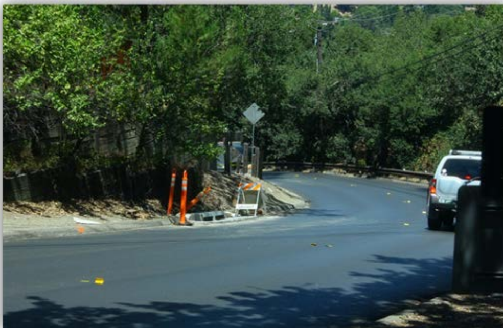
Figure 28: Sight Distance View from Richelle Court #2
