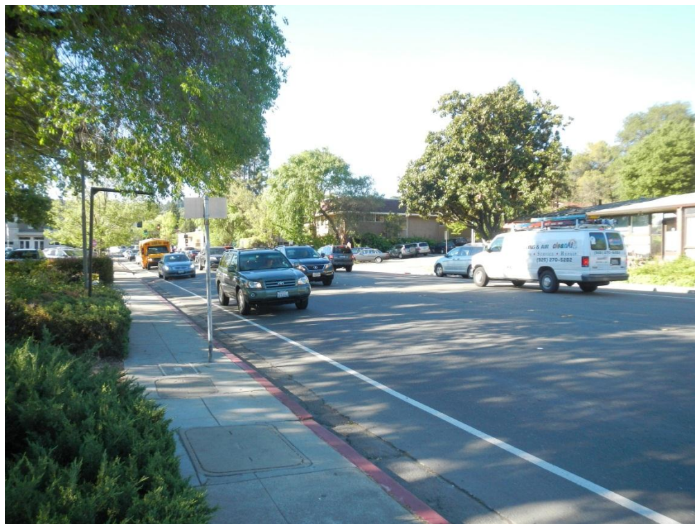
Lafayette Road facing south
