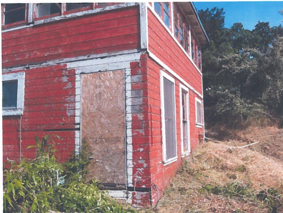
Photograph 6. View looking west of vacant residence at 943 Moraga Road.
