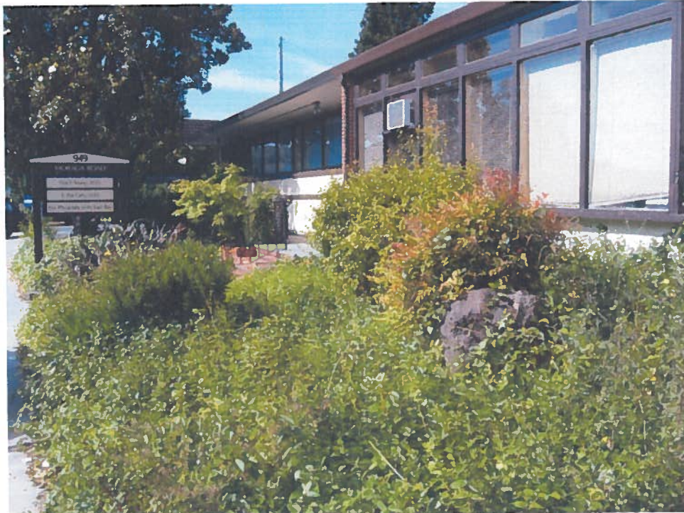
Photograph 5. View looking west of office building at 949 Moraga Road.
