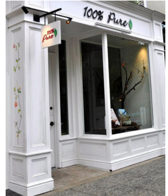
Facade with architectural detailing at storefront
