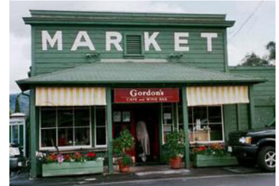
Authentic materials used at upper facade
