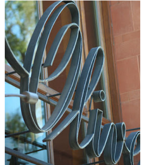
Pinned wall mounted sign at transom level
