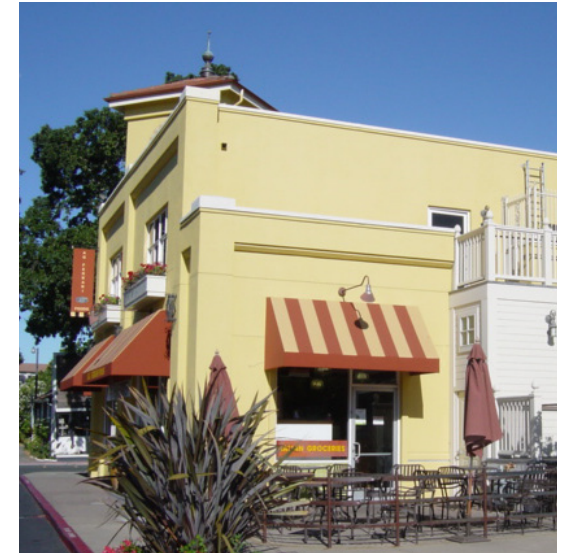
Attention to detailing at side and back of building
