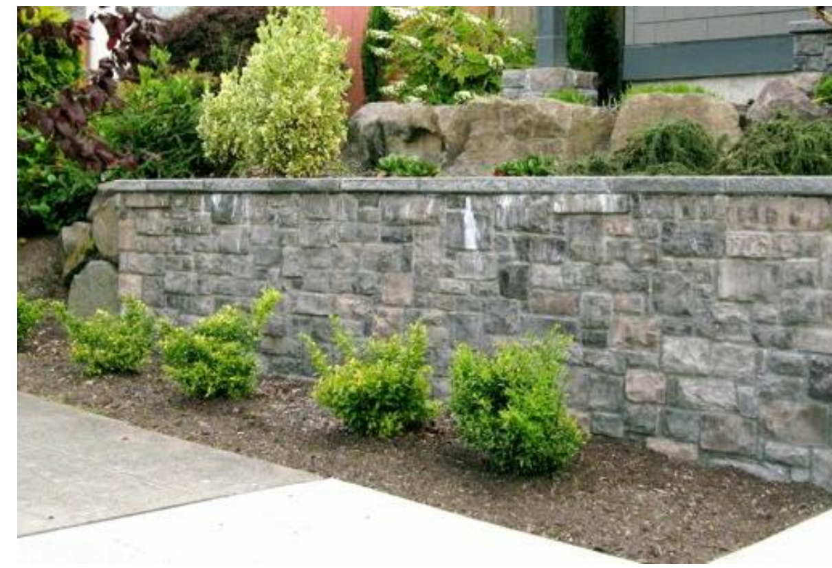
Stone veneer retaining wall
