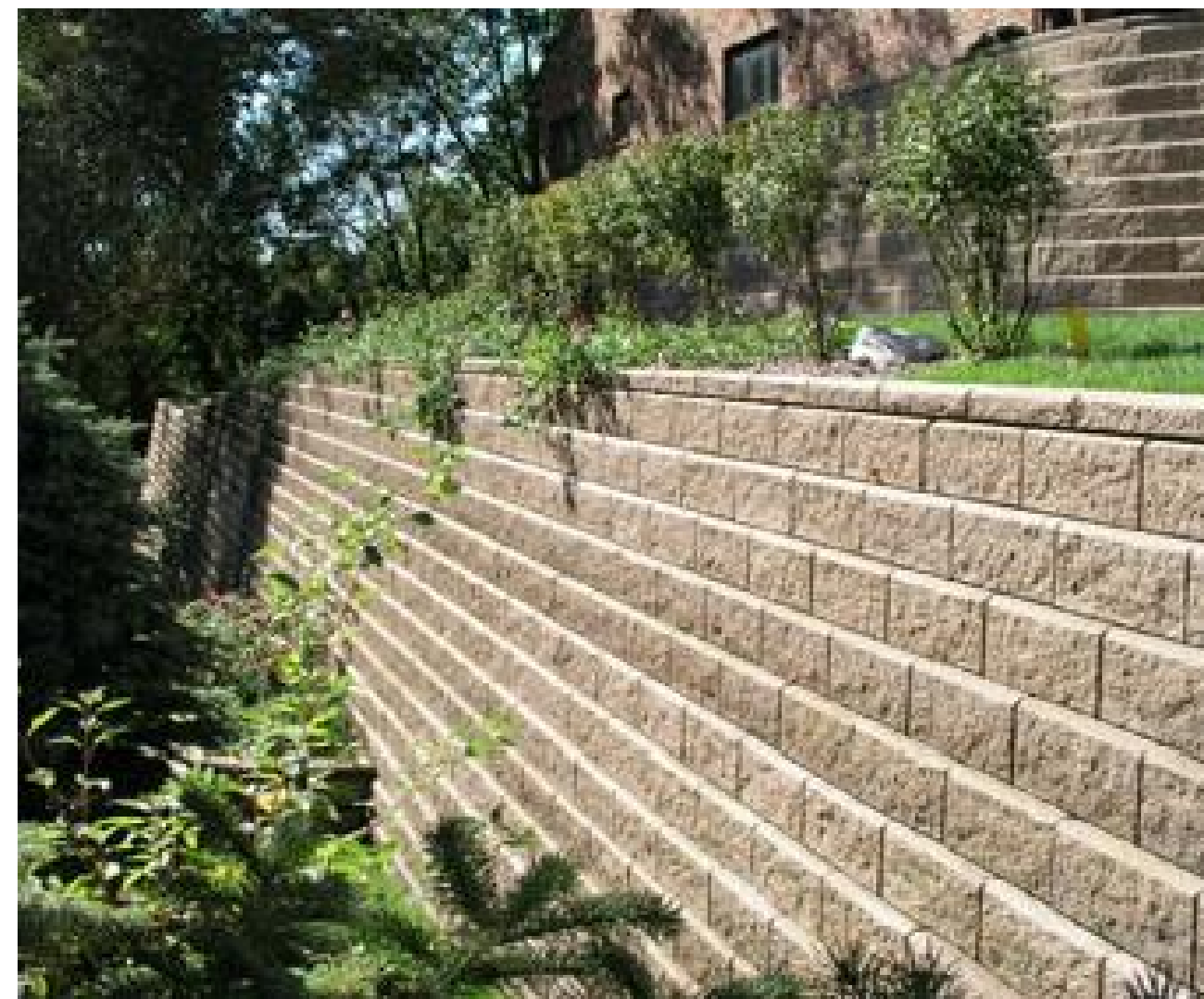
Modular unit retaining wall
