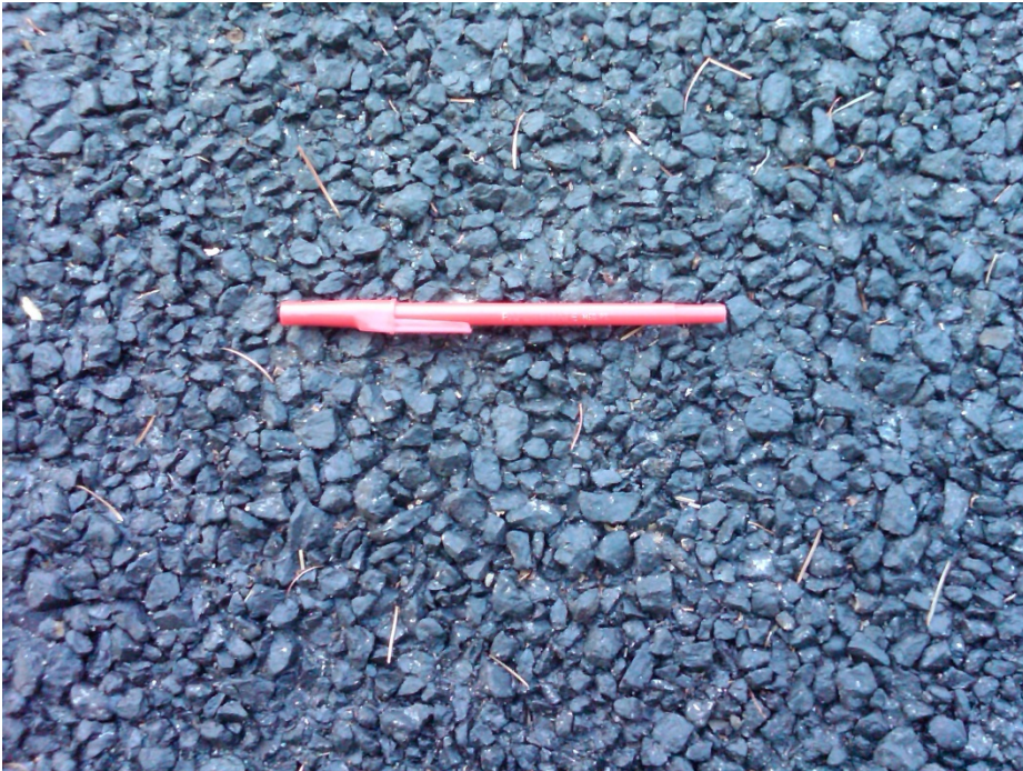
Finished Surface of Pavement with Rubberized Chip Seal
