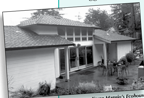
Karen Maggio's Ecohouse operable windows for passive heating and cooling
