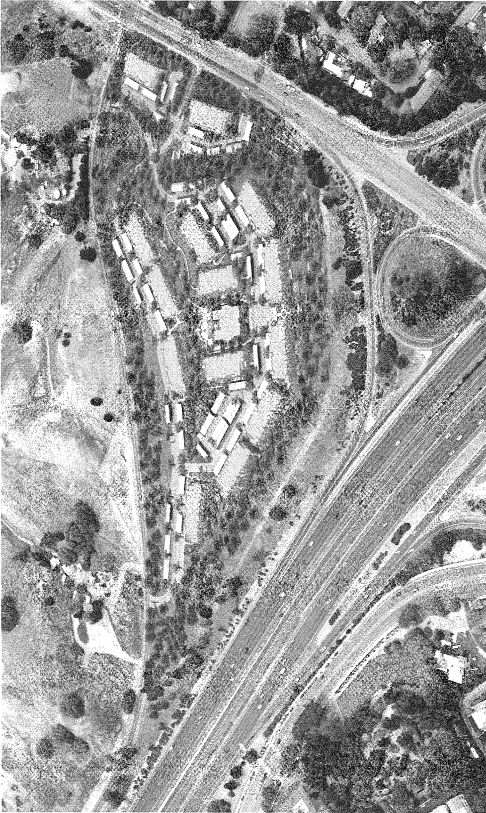
THE TERRACES OF LAFAYETTE APP. 2/27/15-01/27/15 3275 INRAK - 150A - LAFAYETTE, CALIFORNIA 94626 AERIAL SIMULATION (LOOKING WEST)
