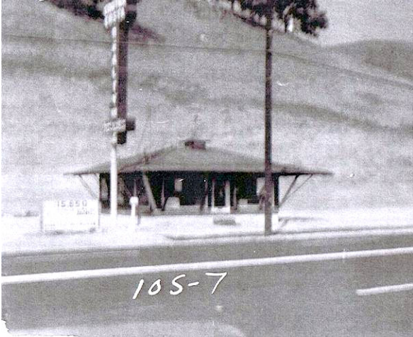
View of the log-faced office building on its original Mt. Diablo Boulevard site, before c. 1965. The building appears to be built on a concrete slab-on-grade and, when moved, raised onto individual footings. Note the angled braces supporting the porch roof, the full-light door, picture windows, vent at the roof's apex and freestanding neon sign. (Contra Costa County. Office of Assessor.)
