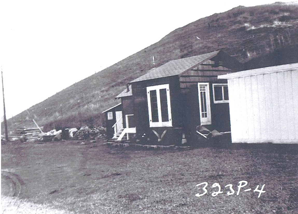
View of the house, during or after 1965. This photograph shows the house before the crawl space was enclosed, the double, single-light doors were replaced by a single, fixed sheet of glass and an awning was installed over the north windows. The shed on the south was removed and replaced by the existing open porch. (Contra Costa County. Office of Assessor.)
