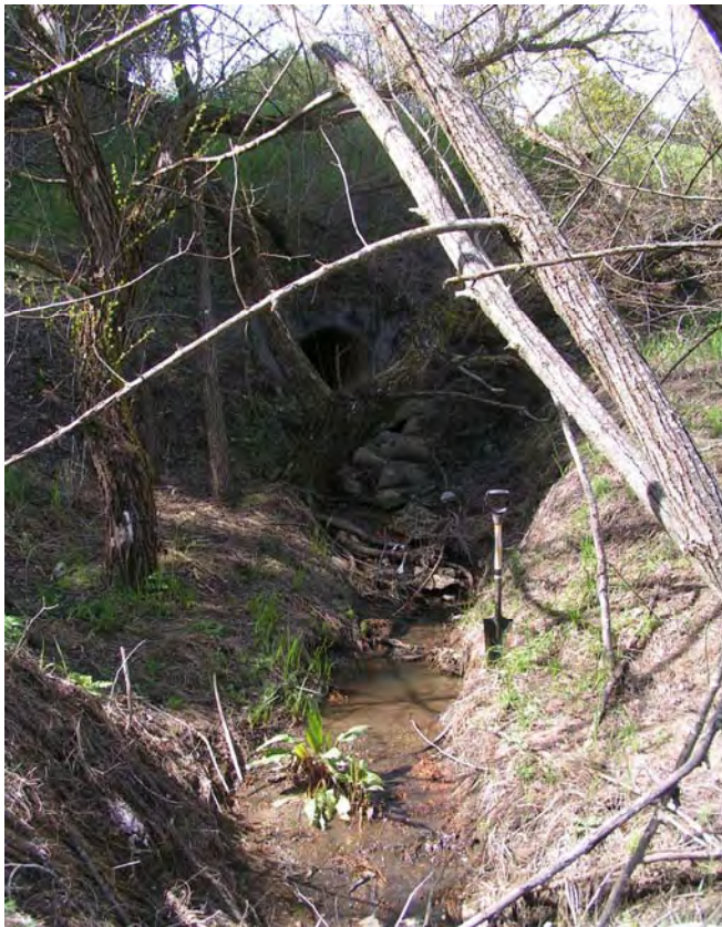
Photograph 6. Location of Transect-3a and 3b, facing northwest (upstream) towards Deer Hill Road (at top of frame above double concrete culvert). The OHWM at this location was approximately 7 feet wide, and the top-of-bank width was approximately 15 feet.
