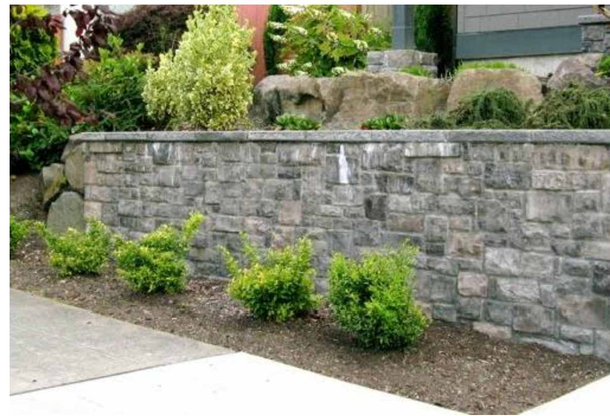
Stone veneer retaining wall
