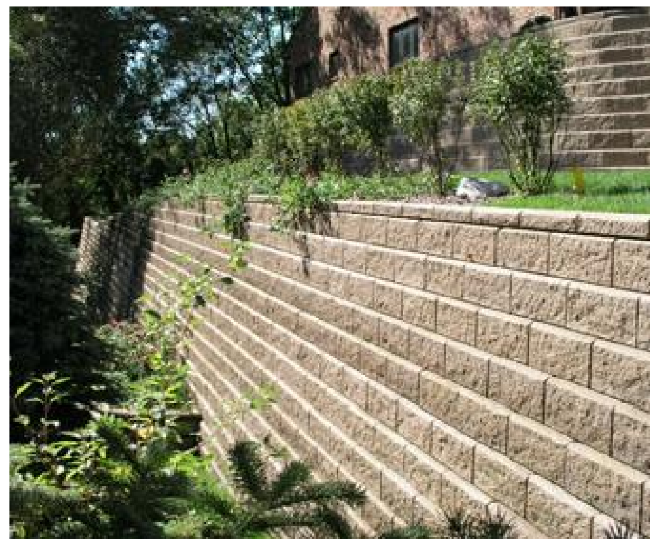
Modular unit retaining wall
